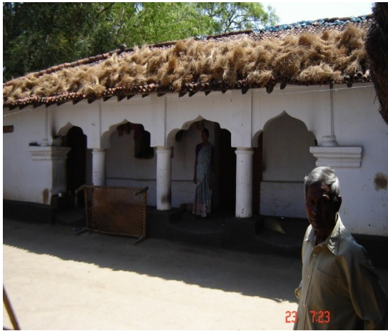
Plate 4 Haus des Dorfpriesters in Jamda: Innenhof
